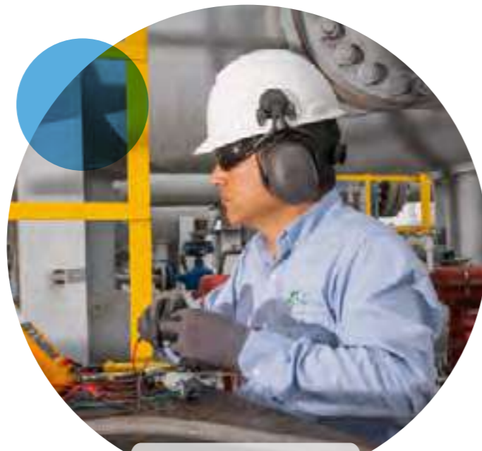
Gas Padua Compression Station Equipment
