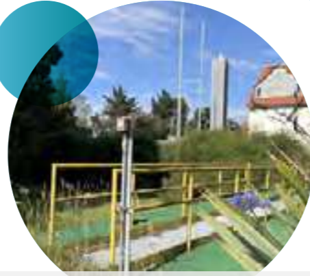
Gas Compression Station La Sabana
